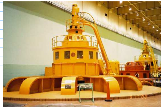
Hydro-Turbine generator
