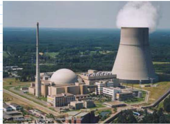
Nuclear Power Plant
