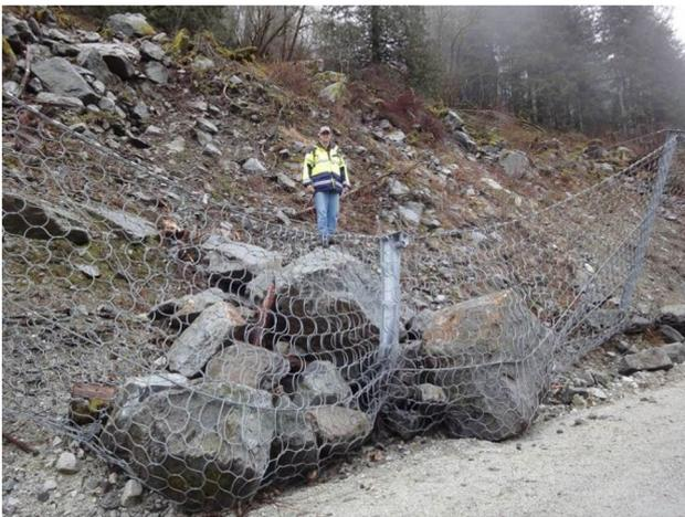
**Fig. 8** Flexible rockfall barrier being impacted by rocks
