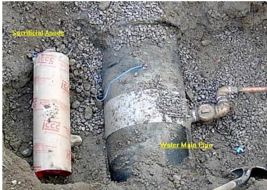
Fig. 11, External cathodic protection of water pipeline by sacrificial anode method
